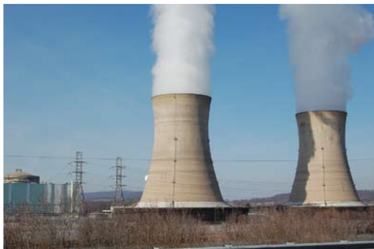
The cooling towers at Three Mile Island (left), a familiar sight around greater Harrisburg.
